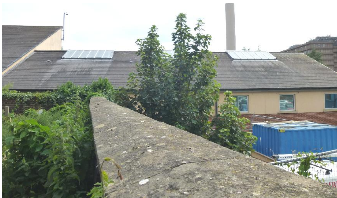
P4: View south west over retaining wall in SW corner.
